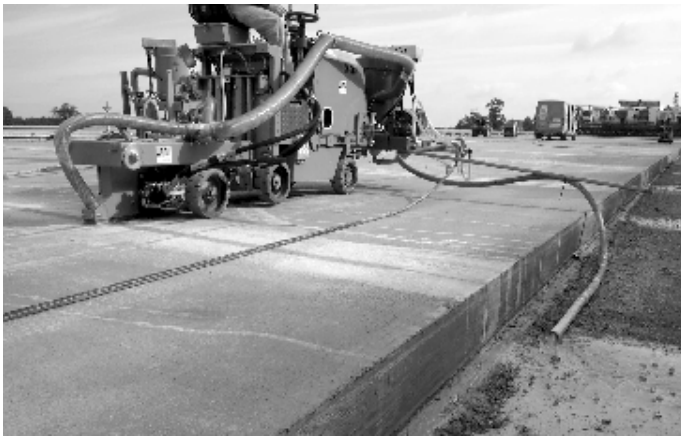
Fig. 11: Modern joint cutter which extracts the mud directly at the saw blade
