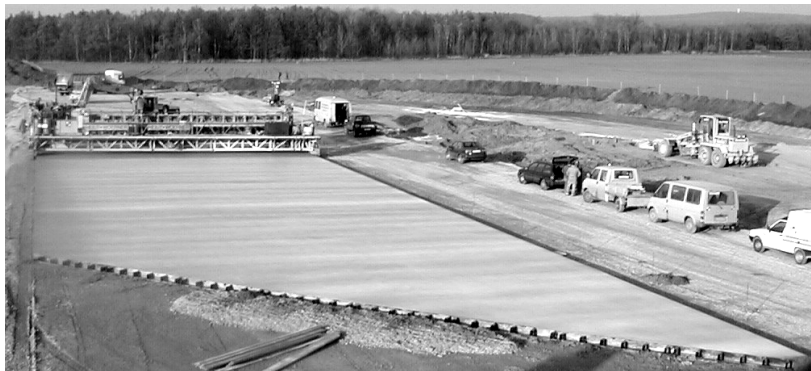
Fig. 6: With special slipform pavers placement width up to 18 m are possible
